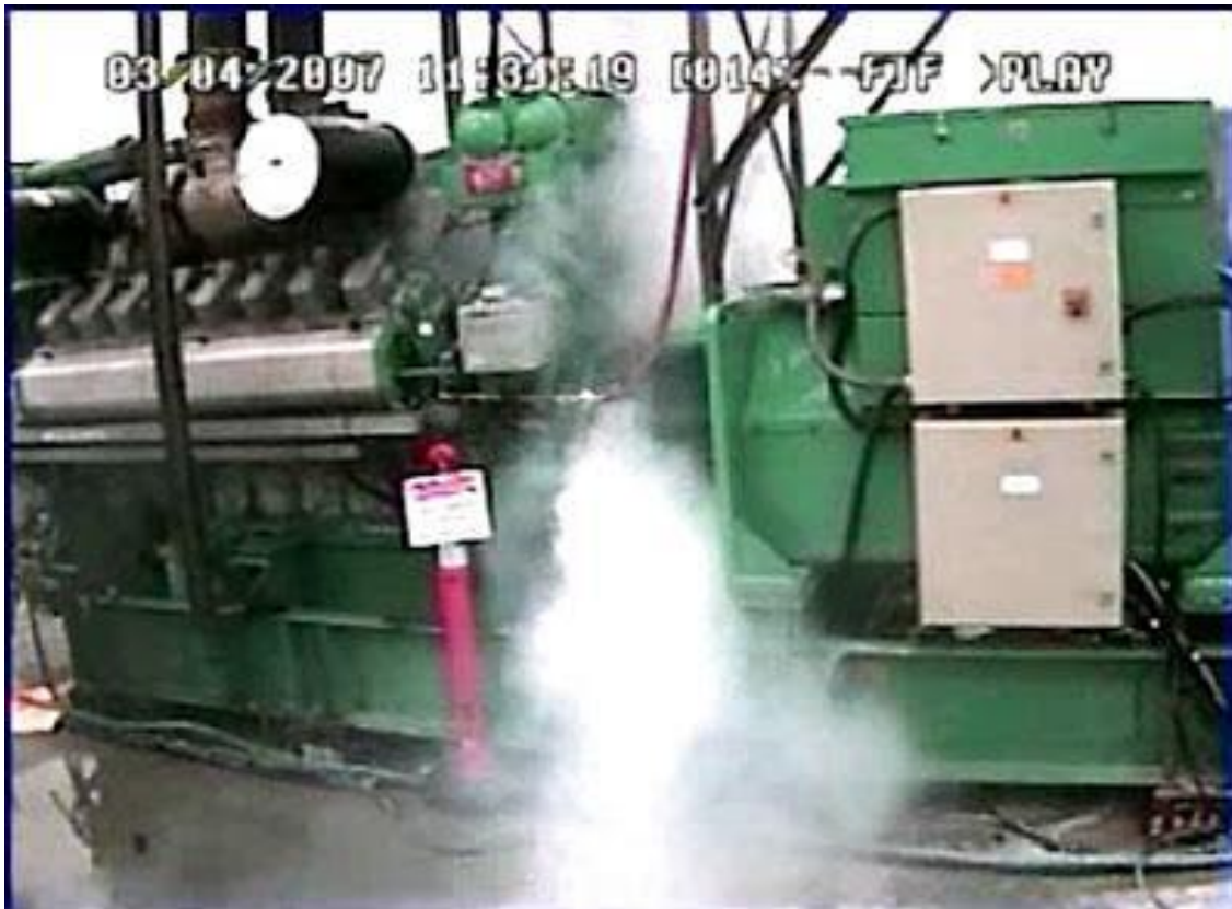
Image 1 - Destruction of a 2.25 Megawatt Generator by Cyber-Attack
