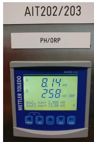
Figure 7: AIT202 analogue output Min/Max values of the pH device
