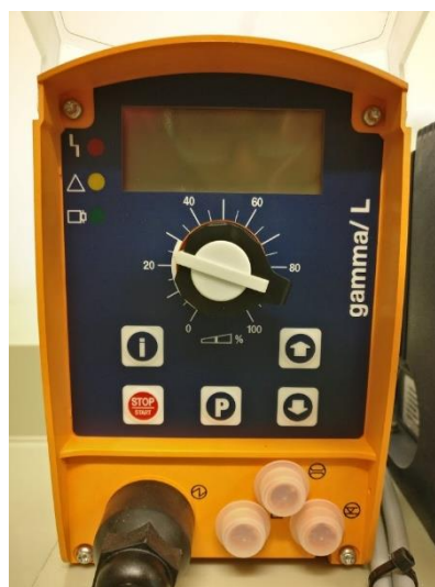
Figure 17: Metering Pump of P205
