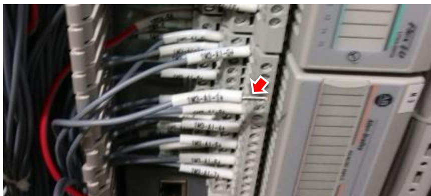
Figure 12: Disconnected AI/O pin
