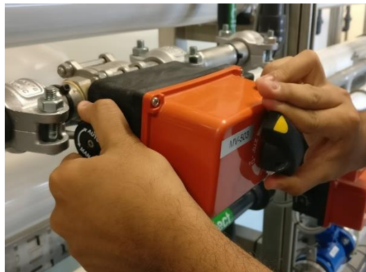
Figure 2: Changing the motorised valve to manual operation mode
